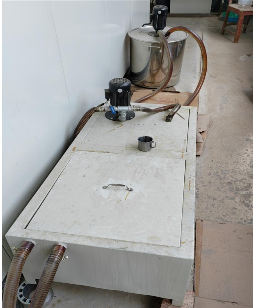
浸漆槽加盖密闭
